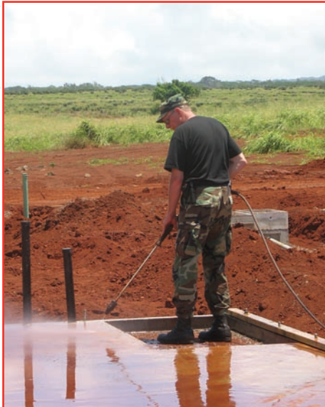
Master Sgt. Melvin Kurtz, Structures Shop, uses a pressure washer to clean a concrete pad at the 'Aloha Gardens' compound.
