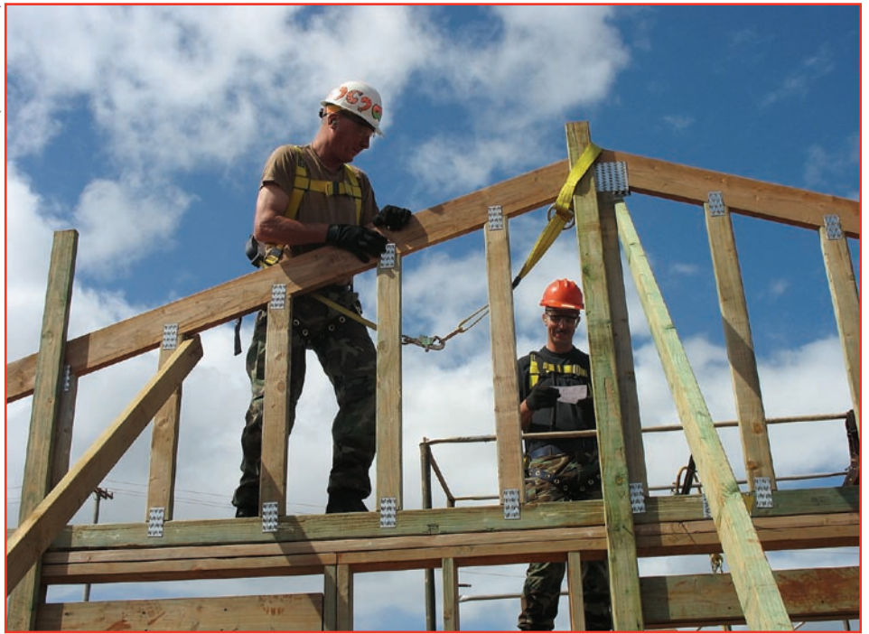
Senior Master Sgt. John Lough, Heavy Equipment Operator, and Tech. Sgt. Steve Tracey, Power Production, work on framing one of the living structures at the 'Aloha Gardens' compound.
