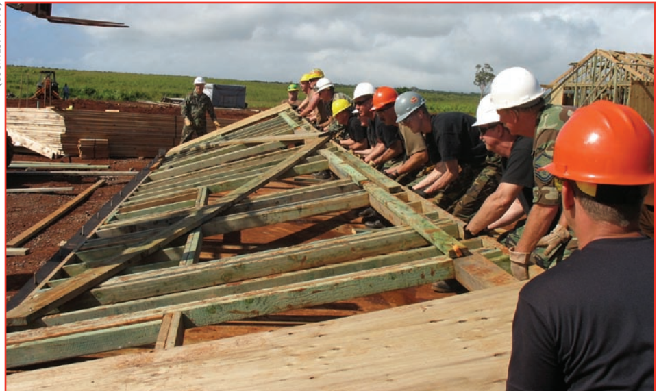
Members with the first rotation of the 931st CES team up to lift part of a frame into place. The 931st CES took part in the Innovative Readiness Project from April 29 to May 28.
