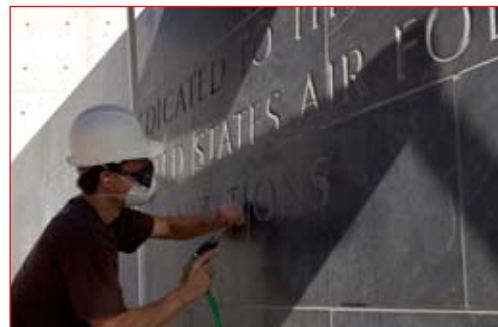
Contractor Marcel Machler chisels lettering at the Air Force memorial being built in Arlington, Va.. The memorial will be complete in October. (U.S. Air Force photo/Tech. Sgt. Cohen A. Young)
